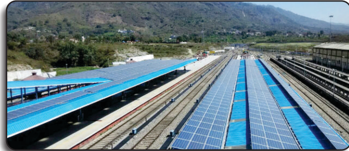
1 MWp SPV Power pack on platform at Shri Mata Vaishno Devi Katra Railway station
